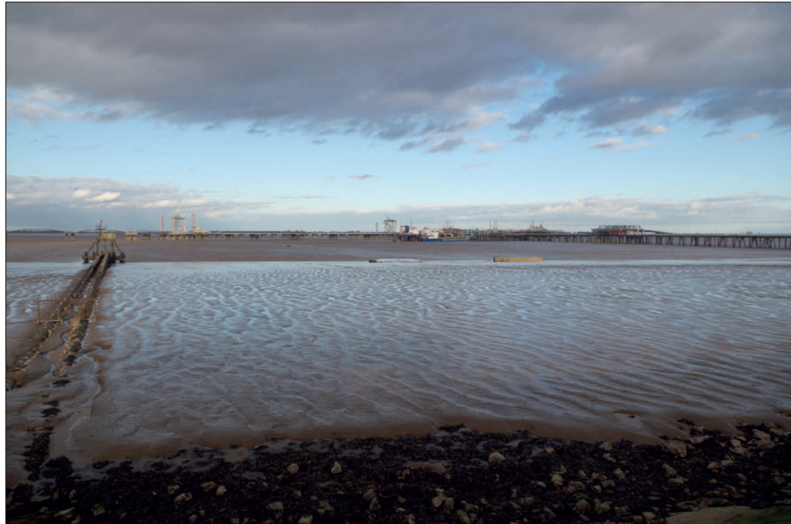
Obstructions 2002 and 2005, as seen from the revetment
