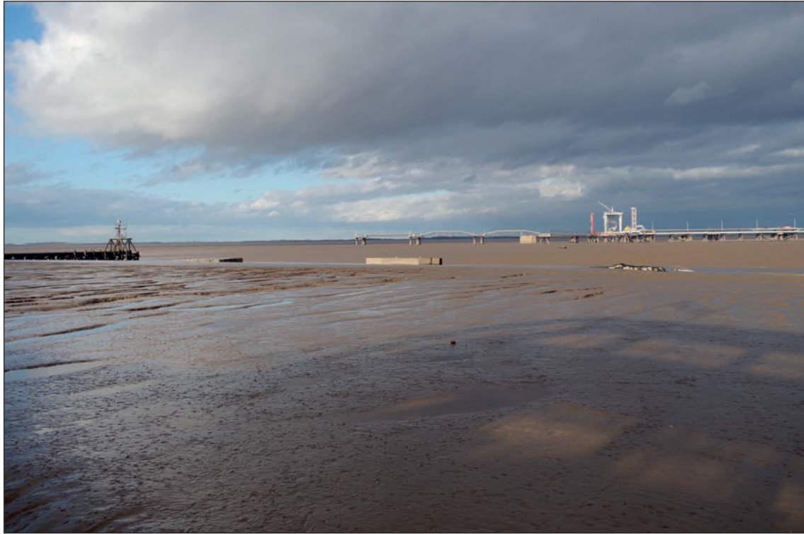
Obstructions 2002, 2005 and 2007, as seen from the revetment
